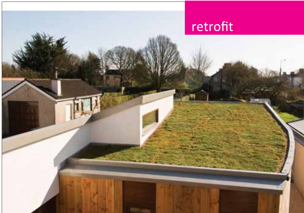
(above) The sedum roof sits on the western side of the extension and is flanked on the eastern side by a pitched roof rising from east to west; (opposite) large sliding doors blur the lines between interior and exterior spaces
